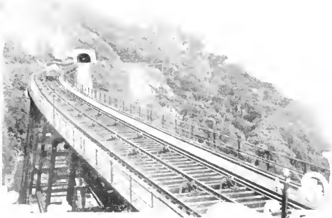
Viaduct on São Paulo Railway.
